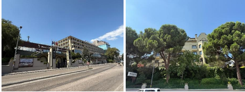
Figure 2. The old and new buildings of Hotel Çelik Palace views
